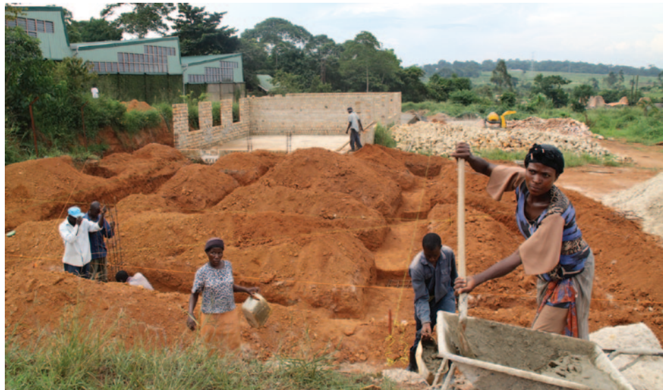
Local builders working on the foundation of the secondary school
